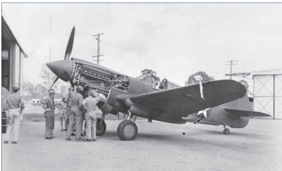
Assembling a United States Army Air Corps P40E aircraft at Archerfield, Queensland, Australia. Photo: Australian War Memorial
