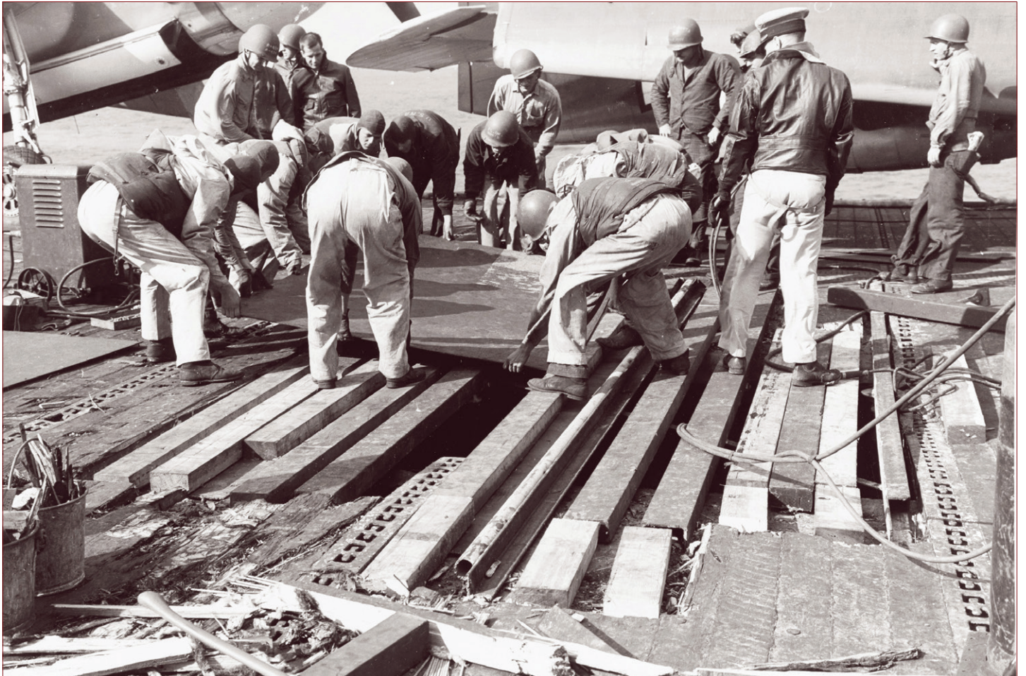
Flight deck of USS Langley (CVL-27) under repair after being hit by a kamikaze, off Formosa, 21 January 1945. Photo: US Naval Heritage Command
