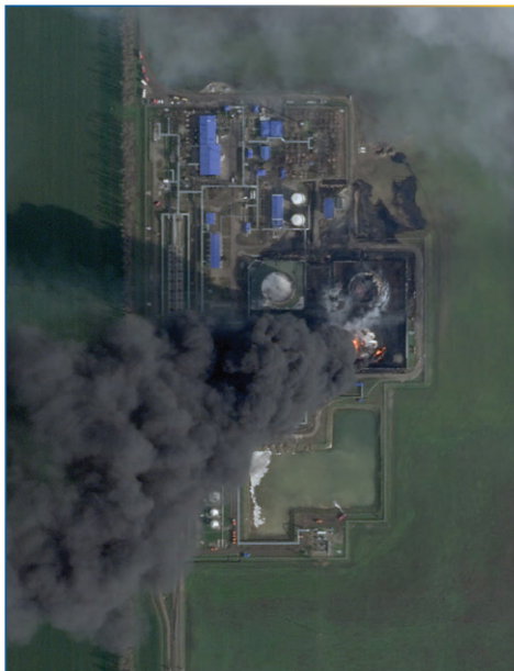
A burning fuel depot in Kavkazskaya as seen in satellite imagery from Planet Labs PBC.
