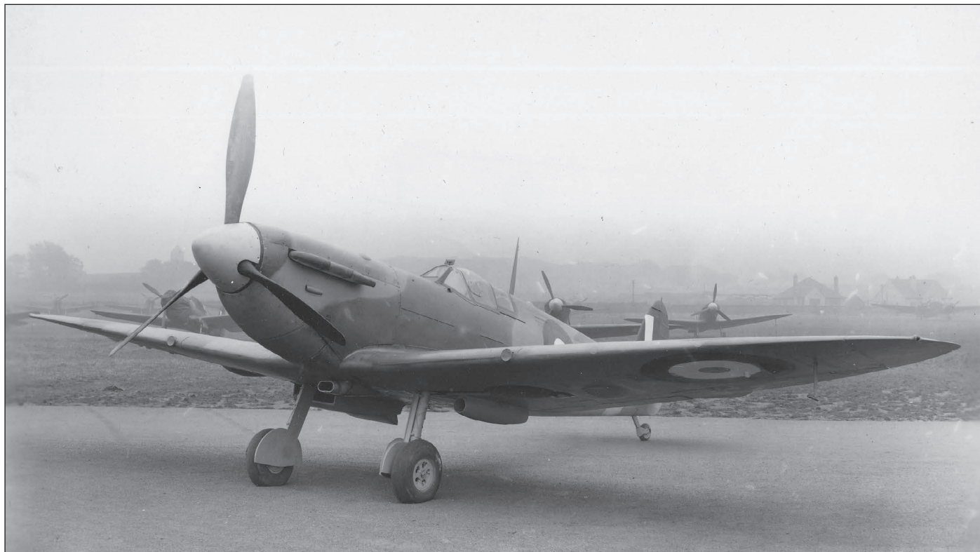
Early production Spitfire Mk.V manufactured in October 1941 with symmetrical lower bulges under the cannon well, enlarged cooler, older canopy style with exterior armor and hinged window hatch. The aircraft still lacks the armament, it's equipped with the De Havilland propeller and newer type of radio Tr.1133 (photo: Simon Erland).
