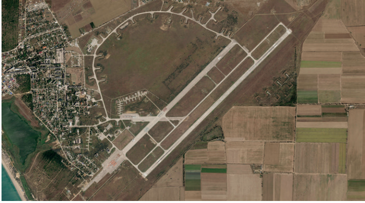
The overall photograph of Saki airport in the morning of August 8 before the attack taken by Planet Labs PBC company.
