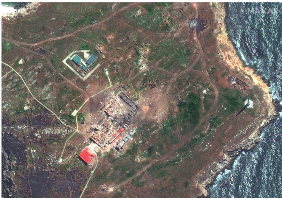
The buildings in the center of Snake Island were destroyed by Su-25s' raid.
