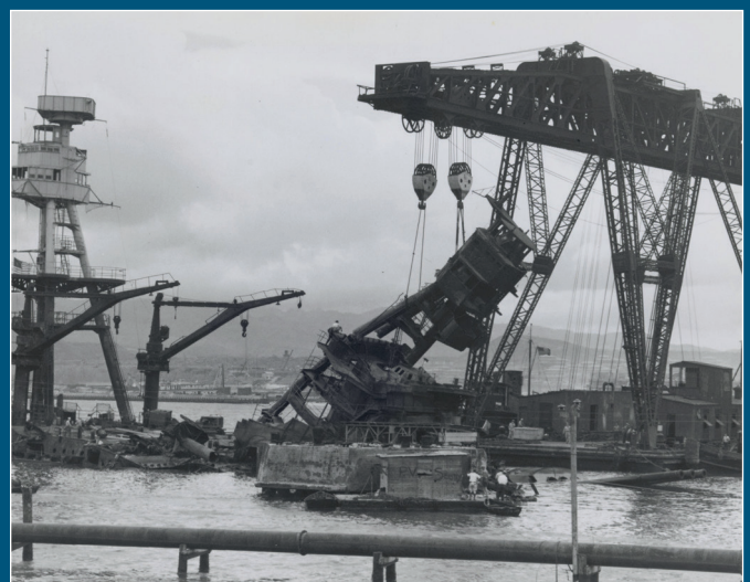
On May 6, 1942, the upper section of the forward mast was cut off the bottom section and removed. The floating gantry crane YD-25, capable of lifting 150 tons, used for dismantling the heavy ship components, served at Pearl Harbor since 1903 (photo: Digital Archives of Hawai'i).
