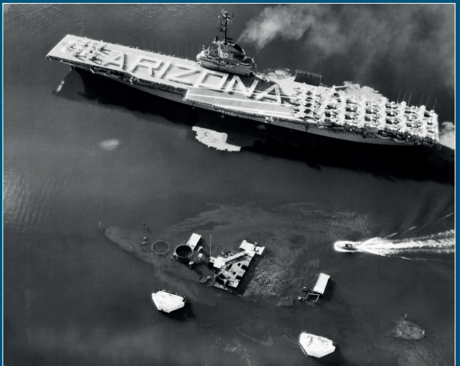
The final wreck appearance after salvage work was completed and her condition in the end of 1950s before the USS Arizona memorial construction started can be seen in this aerial picture taken on Memorial Day, May 31, 1958. USS Bennington (CVA-20) passes the wreck of USS Arizona in Pearl Harbor, Hawaii, on Memorial Day, 31 May 1958. Bennington's crew formed the name Arizona on the flight deck in a tribute to ship's crewmen lost during the Japanese attack on Pearl Harbor. Note the outline of Arizona's hull and oil spillage from her fuel tanks (photo: National Archives).
