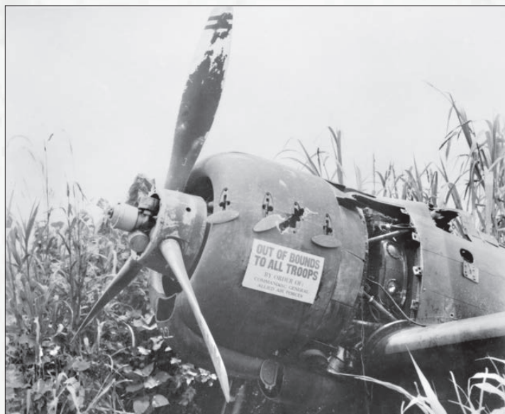
This wrecked A6M2 aircraft found in March 1944 by a reconnaissance patrol on Gasmata airstrip, New Britain was labelled "out of bounds to all troops by order of Commanding General Allied Air Forces" to discourage souvenir hunters. Note the aluminium paint peeling off propeller blade, showing red-brown primer color.
