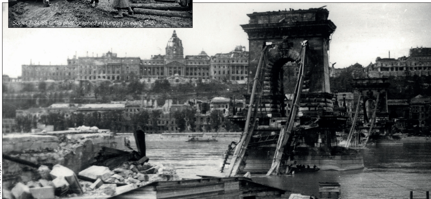
The blasted Budapest Széchenyi Chain Bridge photographed in 1945. The bridge was blown up on January 18, 1945 by the retreating Germans. It was rebuilt, and reopened in 1949. The bridge was designed by English engineer William Tierney Clark in 1839.
