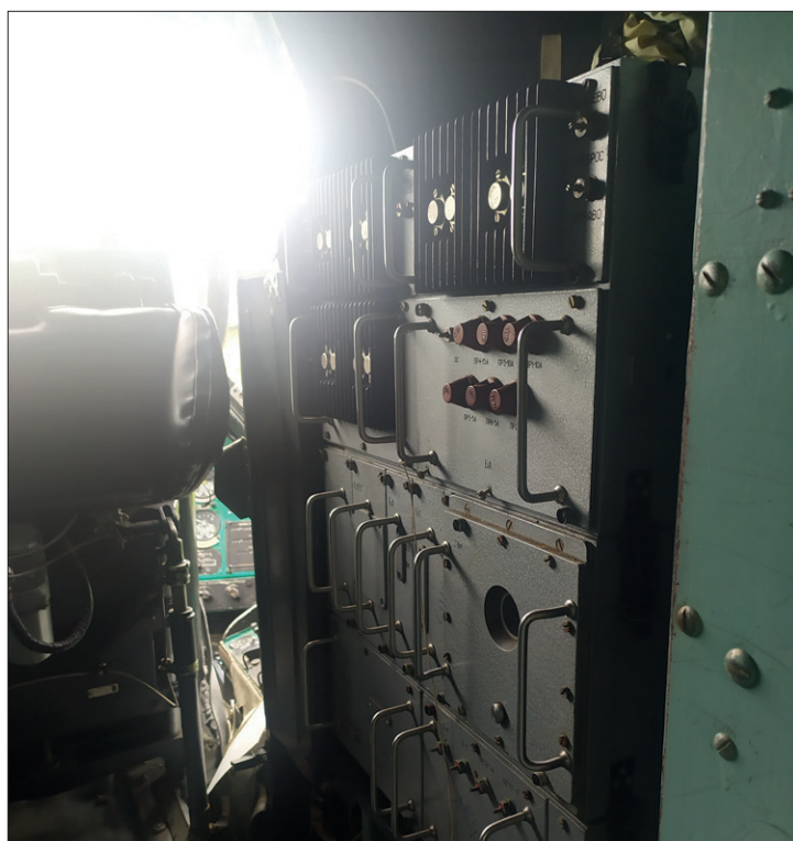
„Hi-fi“ tower, as called, the right side in the tunnel between the cockpit and the D version cargo hold is shown here.
