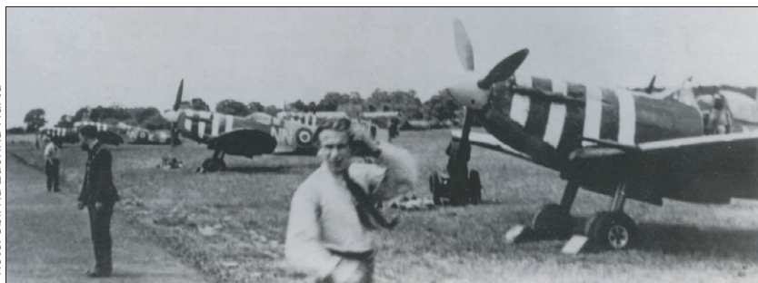
Spitfires Mk. Vb of No. 310 Squadron at Redhill airport in the beginning of June 1942. Noses of all Spitfires are marked by quick identification white stripes. The propeller spinners of No. 310 Squadron Spitfires remained in Sky color, contrary to the official orders.
