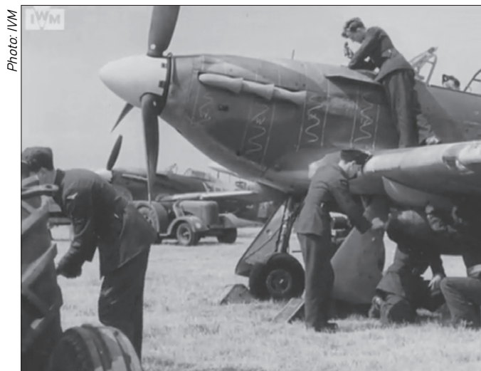
This photo shows, how were the identification stripes painted. Personnel first drew their outlines in chalk, as seen on this Hurricane XP-P from No. 318 (Polish) Squadron.
