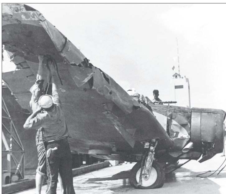
Wreck of dive bomber D3A "Val" from aircraft carrier Kaga. Anti-aircraft defense blew off the rear of the fuselage and dive bomber crashed next to the destroyer USS Montgomery.
