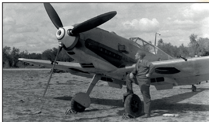
Source: Hanns-Wolrad Dölling via Erik Mombeeck coll. A front view of Bf 109 E-3 6•111 reveals the modified finish of the propeller spinner, whose main part is now painted white, with a red ring added near the tip. The propeller backplate remained in RLM 63, whilst the blades had a standard RLM 70 finish. The decals with the triangular VDM logos, which may be spotted on the earlier picture of 6•111, had apparently worn out.
