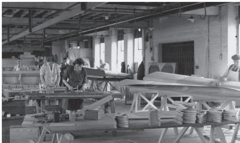
Many female operatives worked in Britain's war industry, and here we can see the Mosquito's wooden components being produced in a manufacturing hall.
