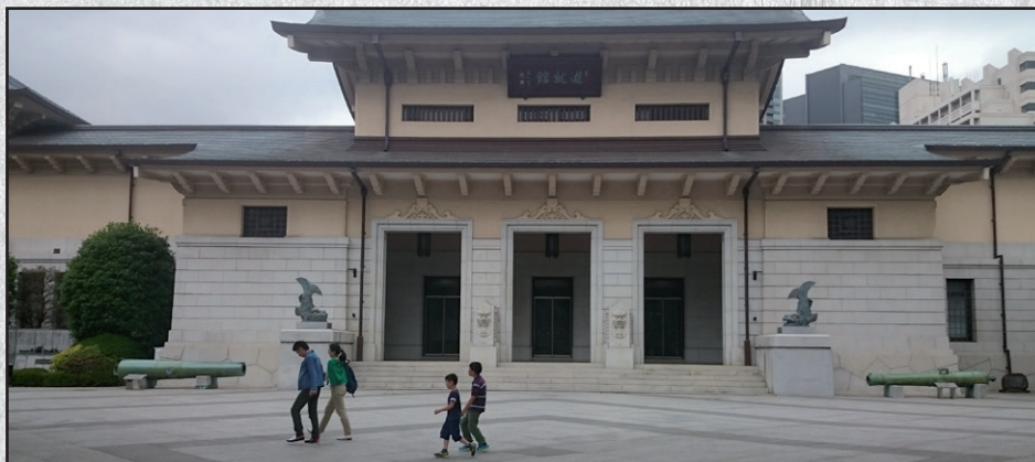
Historical building housing the Yūshūkan museum.
