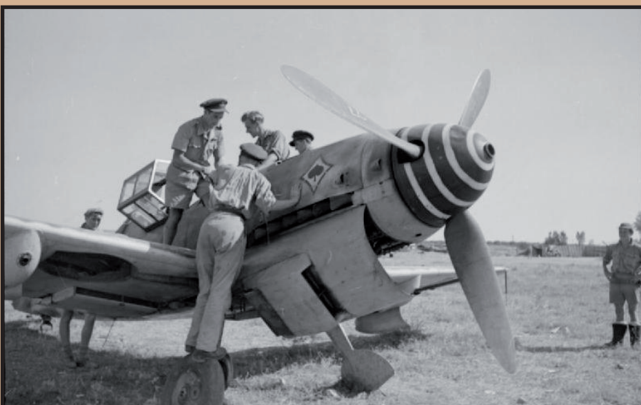
Curious members of No.43 Sq RAF examine an abandoned Bf 109G-6 of 6./JG 53 (II. Gruppe) at the Sicilian base at Comiso. The twin cannon pods and the paired 210mm rocket tubes were common fixtures on aircraft of III./JG 53. In fact, Amon's 7./JG 53 was specialised in the use of rockets against bombers as so-called 'Werferstaffel' over the second half of the year. Within JG 53, III. Gruppe was consequently referred to as 'Schwere Gruppe' (Heavy Group) and in 1943 became the most successful fighter Gruppe in the Mediterranean. (Photo: IWM CNA 1045)
