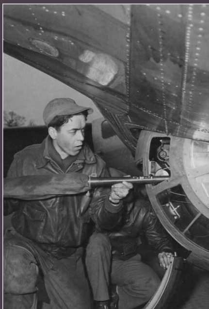
The installation of the M2 in the B-17G ball turret.
