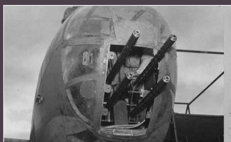
A quartet of M2s in the nose of the B-25 Mitchell.
