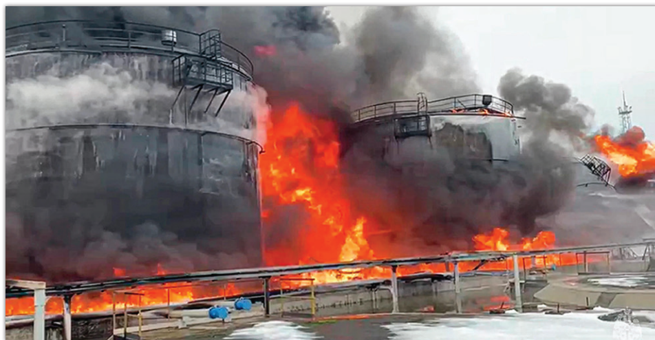
Fire at a fuel storage facility in the Bryansk region. According to the initial report from Russian authorities, there was no damage, and two Ukrainian drones were shot down, likely directly above the fuel tanks.
