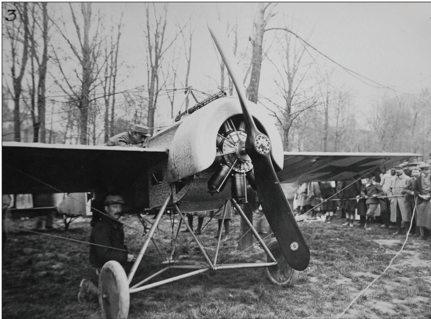
The Fokker was equipped with a Garuda propeller. Photo: National Museum of the U.S. Navy
