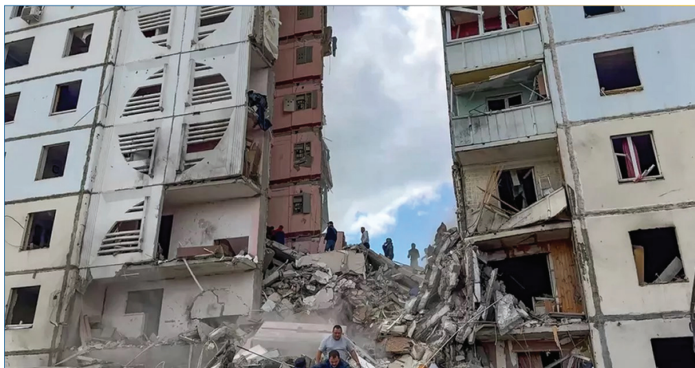
An apartment building destroyed in Belgorod on May 12.
