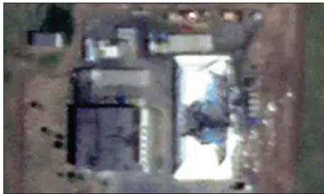
Close-up of a hangar with a broken roof, through which a pair of Su-34s can be seen.
