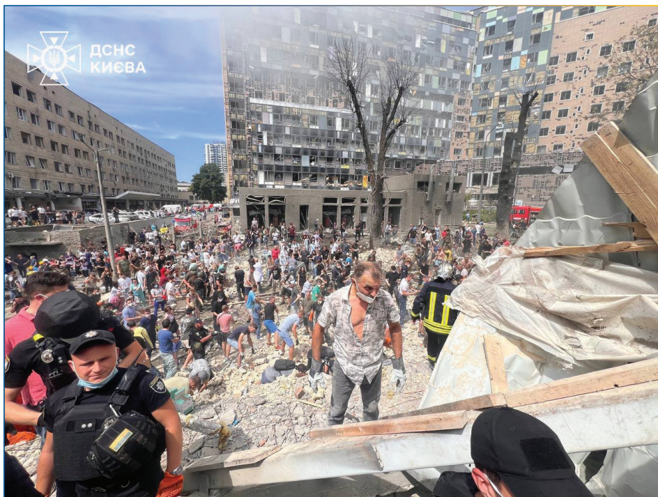
Struck children's hospital Ochmatdyt in Kyiv.
